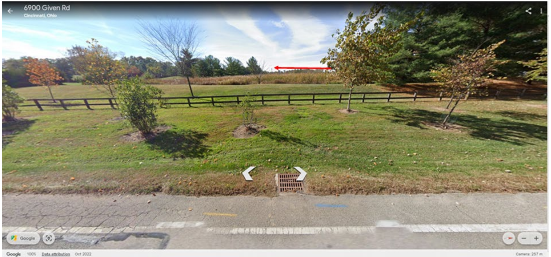
View of Cell Tower From Given Rd.:
